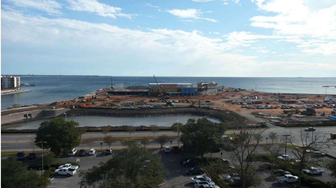
Project Under Construction
