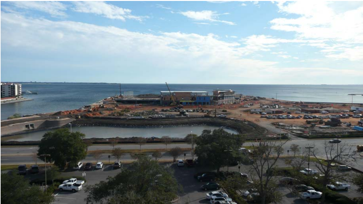
Project Under Construction
