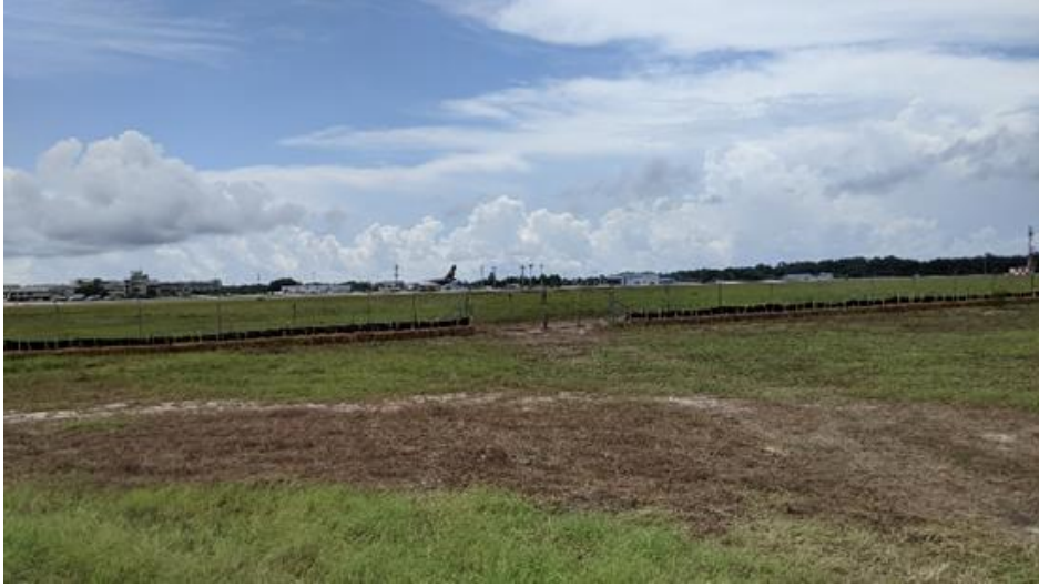
Photo 1.3: Security perimeter fence delineating Airside from Landside. Gate installed to allow authorized individuals onto Airside.
