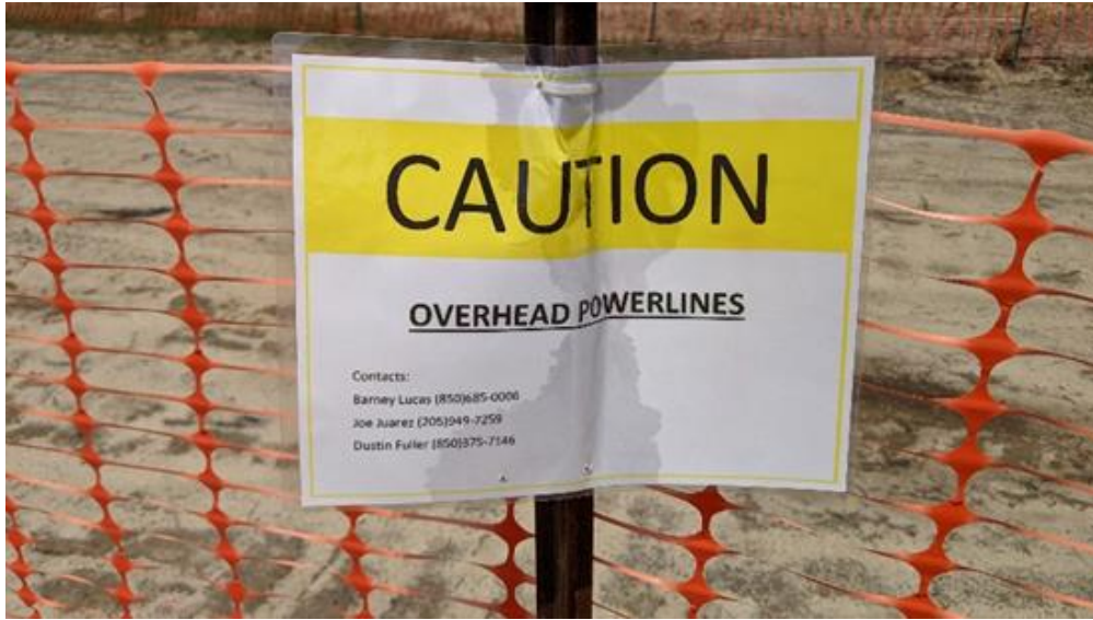
Photo 1.9: Located and identified overhead powerline area with appropriate contact information.
