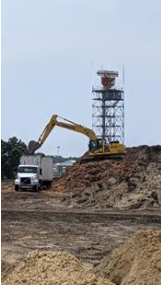
Photo 1.13: Hauling away wood chips from clearing and grubbing operation.
