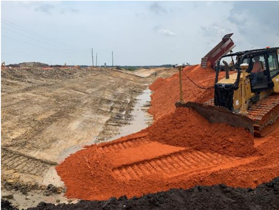
Photo 1.6: Initial bridging of water in existing drainage ditch.
