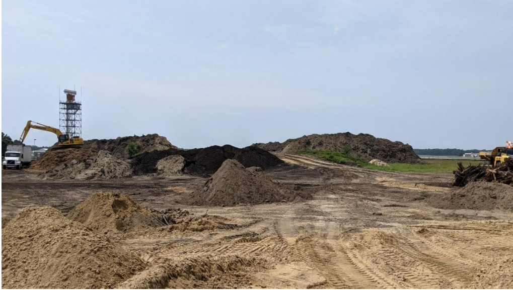
Photo 1.15: Separation of soil types. Topsoil separated from subsoil and sandy suitable backfill material (not shown, located on other side of these piles).
