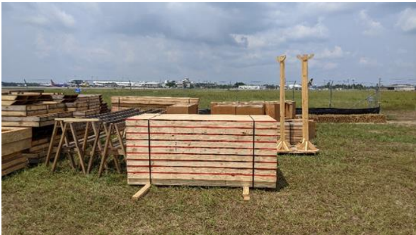
Photo 1.14: Job built concrete forms of various sizes and usages.
